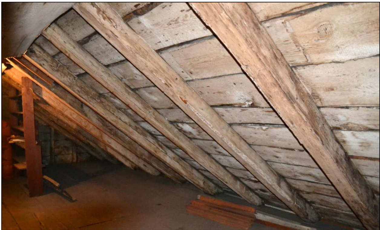
West slope of the roof, looking southwest and showing rafters below the level of the collar ties.
