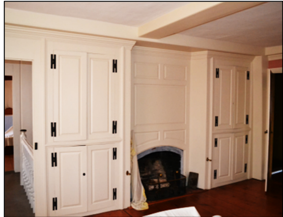
Right: Room 2-3, Northeast chamber, second story; H hinges are reproductions
