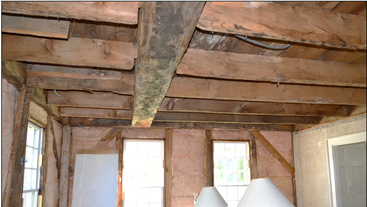
Hall-Dyer second-story frame above the parlor, looking south. Note that the wall post in the southeast corner (left) was hewn back and scarified to receive plaster and thus to be invisible from within the room.
