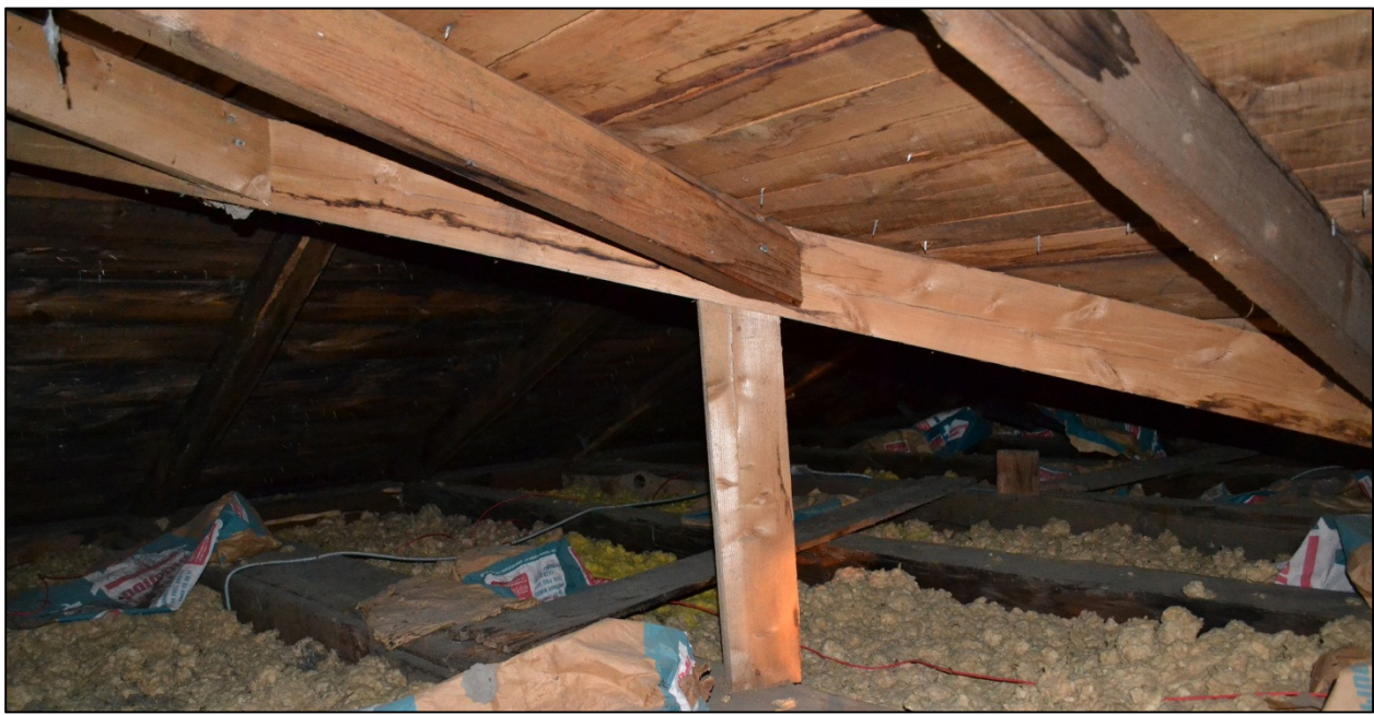
Replaced hip and jack rafters and roof sheathing at the intersection of the roofs of the main house roof and the wing, looking southwest from the attic of the wing toward the main attic.
