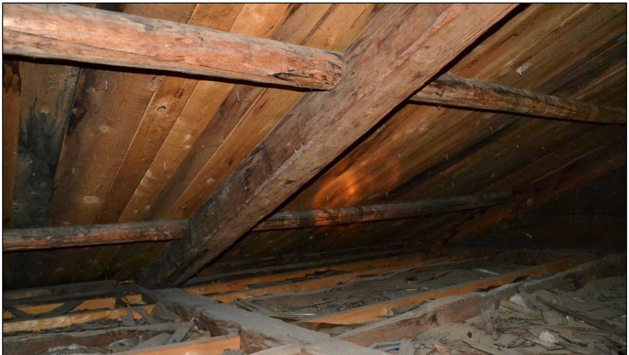
Hall-Dyer House, Tamworth, New Hampshire: Roof frame of added wing, looking northwest, showing a principal rafter and two horizontal purlins. The roof sheathing is modern.
