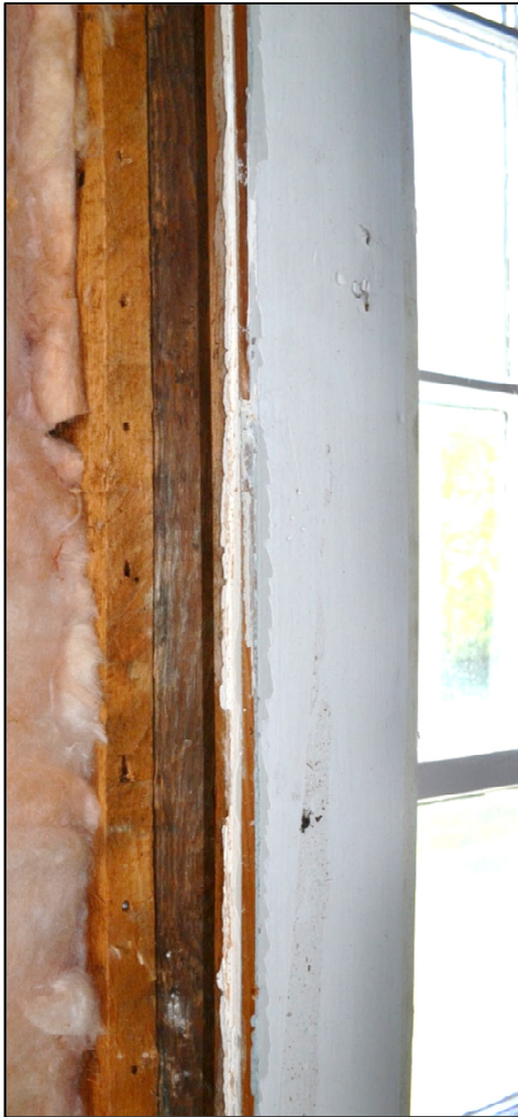
Left: Parlor window, showing a single set of nail holes on the stud for lath
