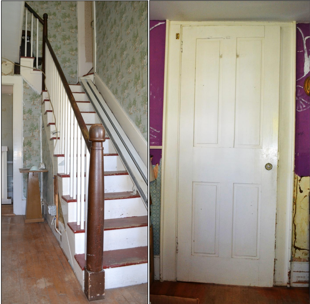
Left: Balustrade in front entry, showing heavy, turned newel and angle posts
