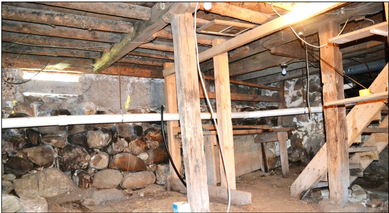
Hall-Dyer basement, looking southwest, showing fieldstone walls and split granite underpinning
