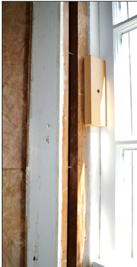
Right: Parlor window, showing a single set of nail holes for the window casing
