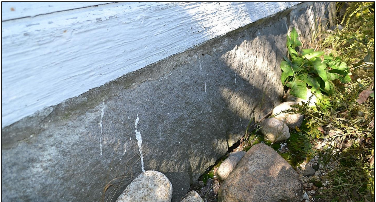
Underpinning stone on the south elevation (façade), showing plug drill holes along bottom edge
