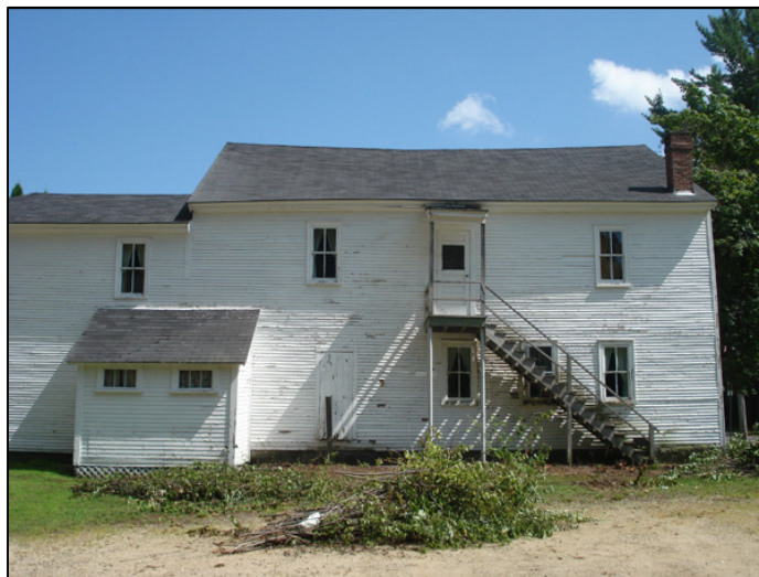
Rear elevation, Moultonborough Grange building, showing distortion of the roof, August 2, 2012. Photo courtesy of Cristina Ashjian.
