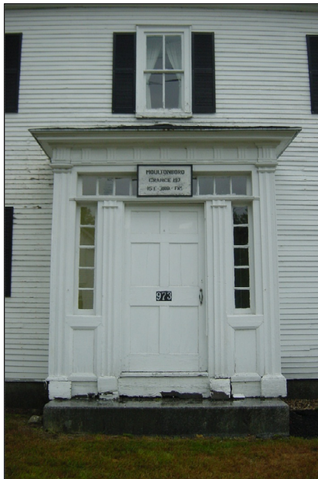
Front entry, displaying a federal-style front door and a Doric entablature.
