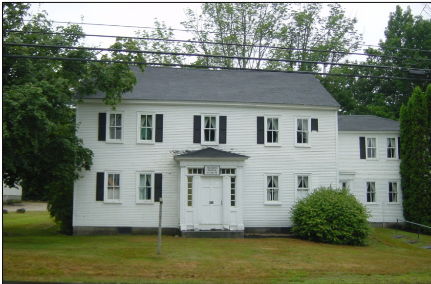
Moultonborough Grange No. 197, looking northwest
