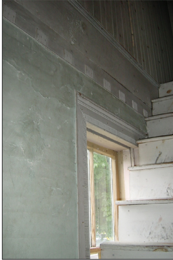
Reeded window casing and entablature with reeded triglyphs in the former parlor on the southwestern side of the building, partly obscured by a staircase leading up to the back of the second-story stage.
