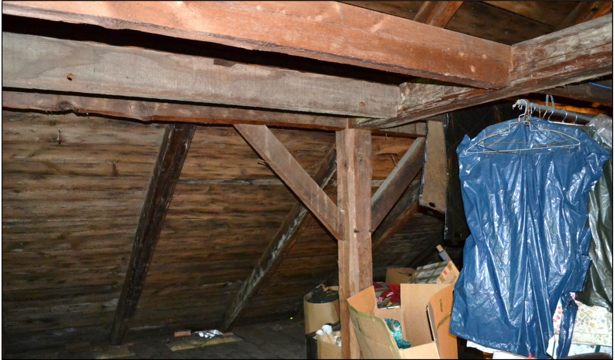
Added roof frame of the Union House Tavern, looking northeast, showing one post of the boxlike supporting framework of the broad roof.
