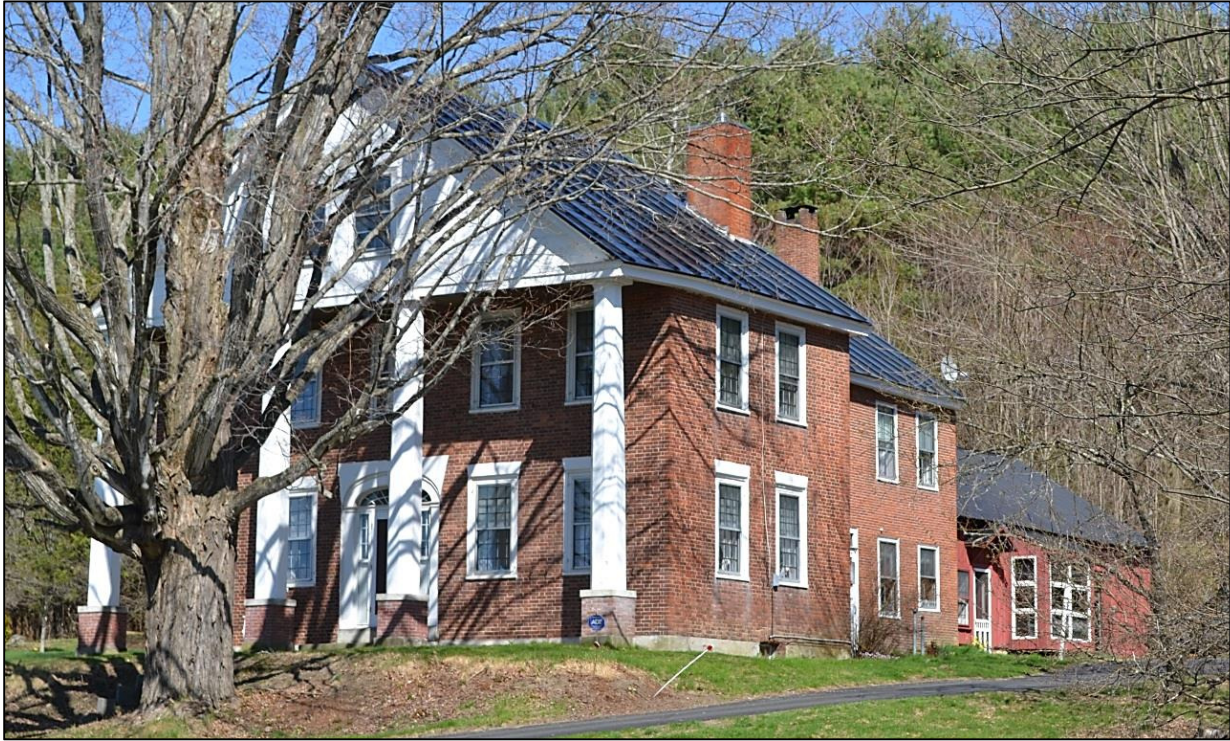
West and south elevations, Union House Tavern, Haverhill, New Hampshire, looking northeast.
