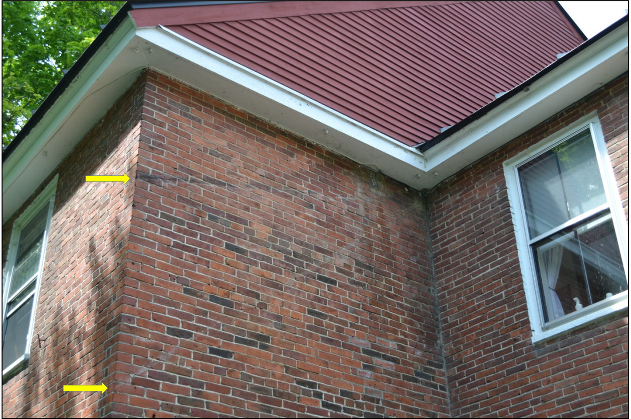
Rear (east) wall of the original Union House (left) and south wall of the added wing (right), looking northwest.
