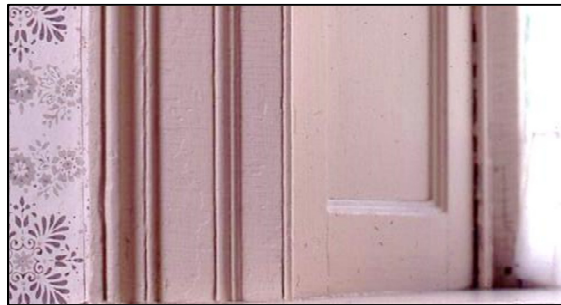
Architrave (window casing) with the same profile, Grafton Hotel (c. 1815), Haverhill Corner
