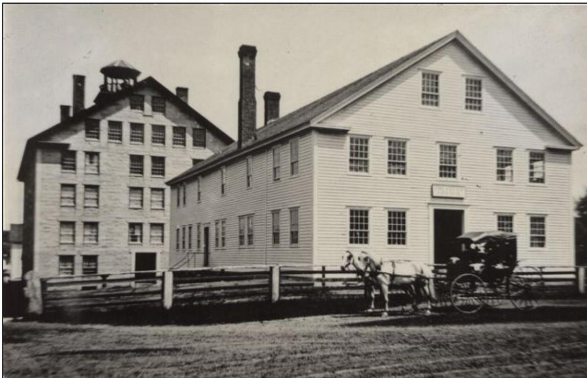
Above: Store building (right) and Great Stone Dwelling (1837-1841), Enfield Shaker Village.
