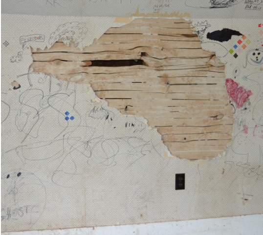
Exposed area of split-board lath
