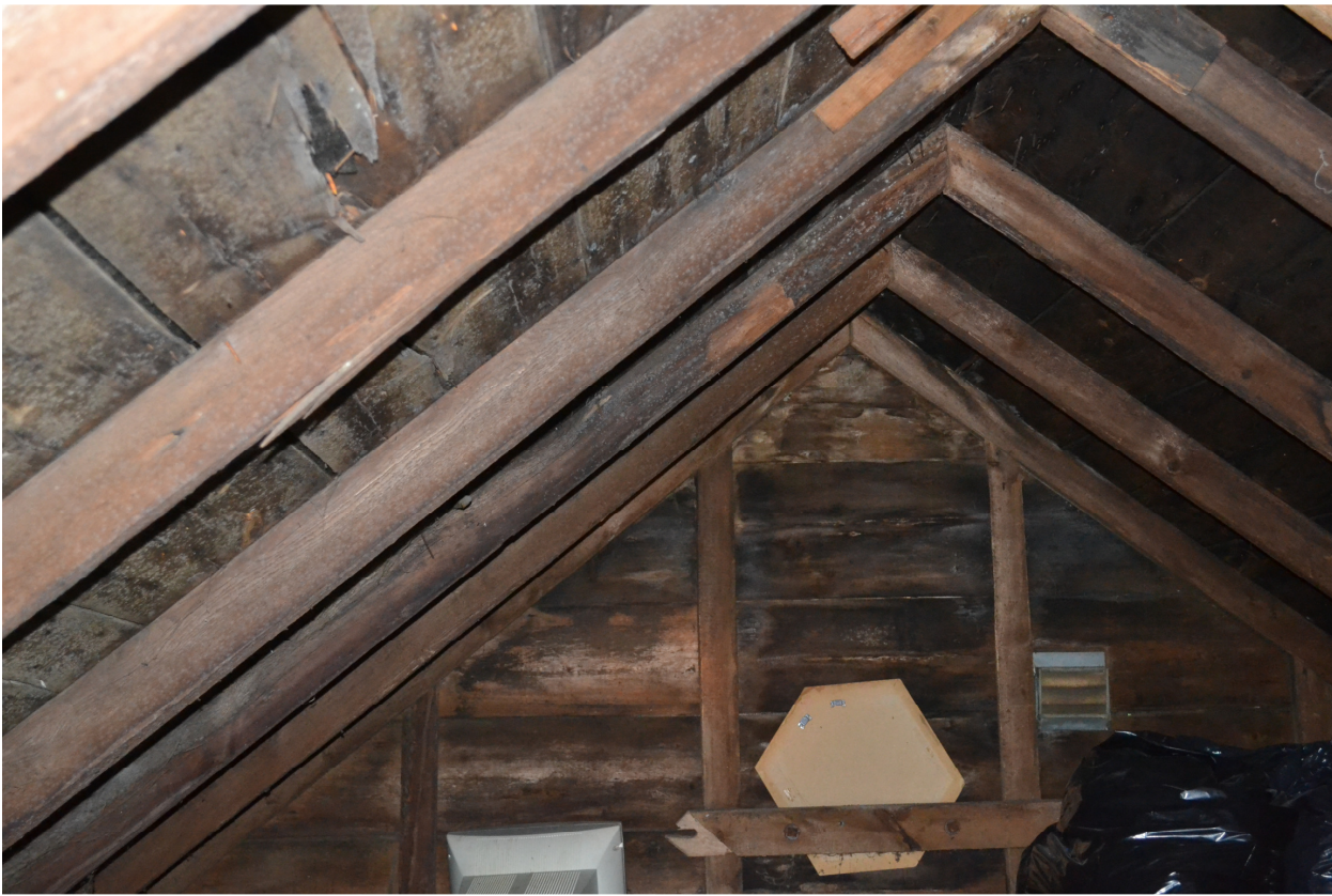
Roof frame of the wing of the Greeley House, with widely-spaced common rafters and no ridgepole.
