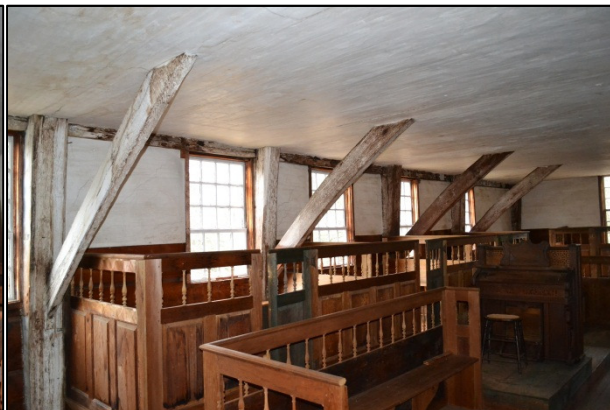
Gallery, looking southwest, showing braces between posts and tie beams (above ceiling)
