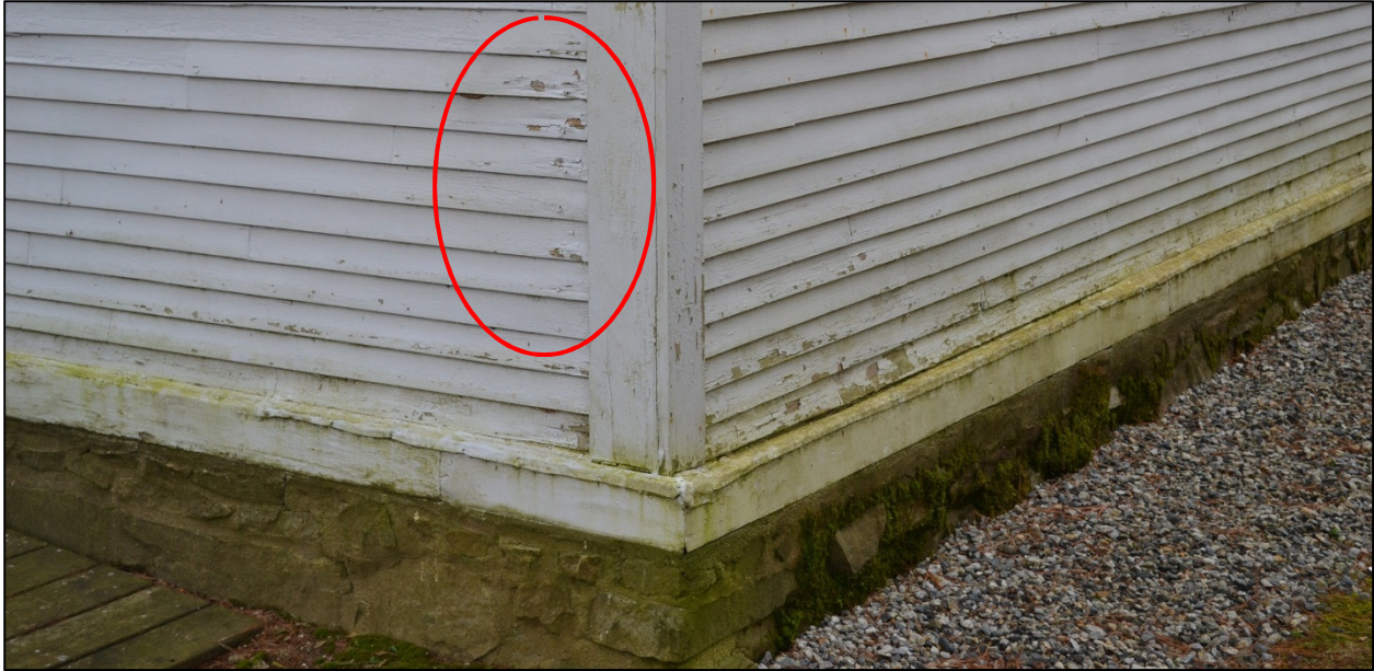
Left: east side of the building, showing deteriorated clapboards at corner; right: rear (north) wall showing algae growth on water table and moss growth on foundation stones.
