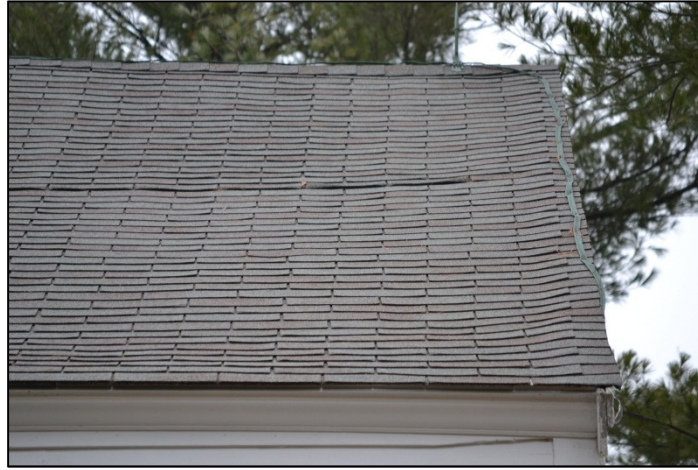
Southeast corner of roof, showing separation of butts at one course of shingles.
