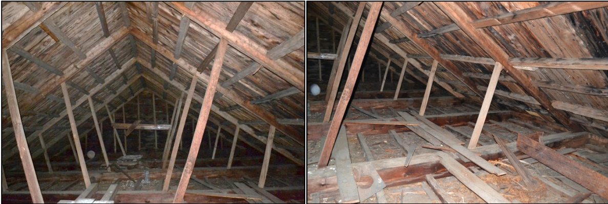
Left: Longitudinal view, looking east. Platforms for two former brick chimneys rest on tie beams at the left of center.
