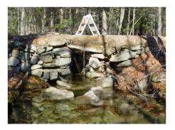
Dry-laid stone box culvert on Gore Road, Warner, N. H., showing minor flood damage. (Photograph by James L. Garvin)
