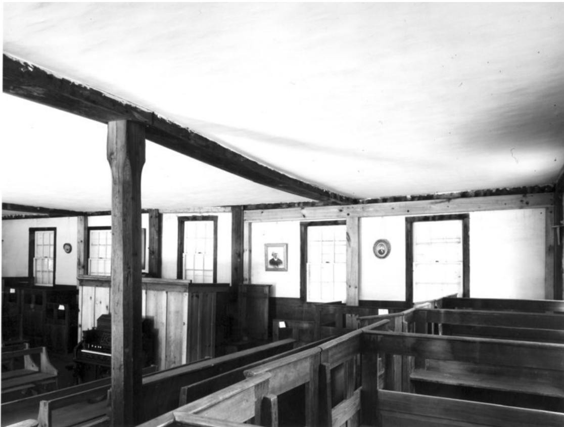
ALLENSTOWN MEETING HOUSE As it appeared before the fire of July 15, 1985 showing the deflection of the truss tie beam from roof loading and weight of the plaster ceiling
