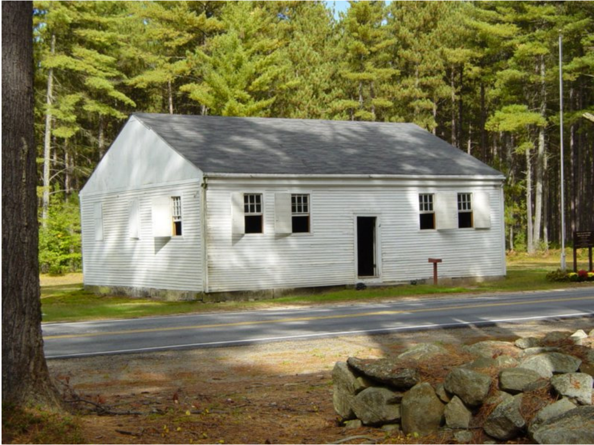
ALLENSTOWN MEETING HOUSE 100 Deerfield Road Allenstown, New Hampshire Prior to replacement of roof in 2006 and re-clapboarding in 2010
